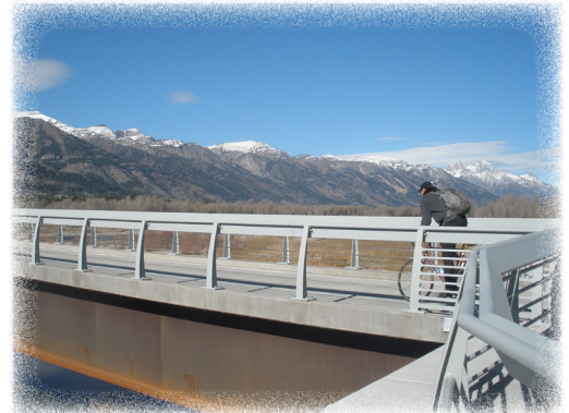
New Snake River bridge, part of the pathway network parallel to WY-22, opened in fall 2014
