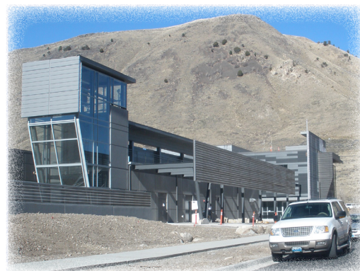
New transit vehicle maintenance facility (phase 1 complete)
